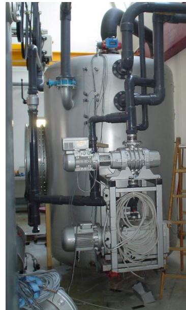
Figure 9 To the left it appears how the pressure and temperature measurements of the compressor performance were made primarily by sensors in the compressor house and partly by a robot on top. To the right it appears how vacuum is maintained by means of a Roots pump and a rotary vane pump.
